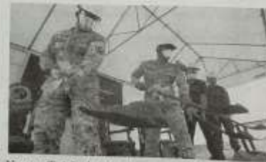
Navy officials break the ground for the first of three new hangars of the Naval Air Wing headquarters in Cavite City, marking the start of construction.
